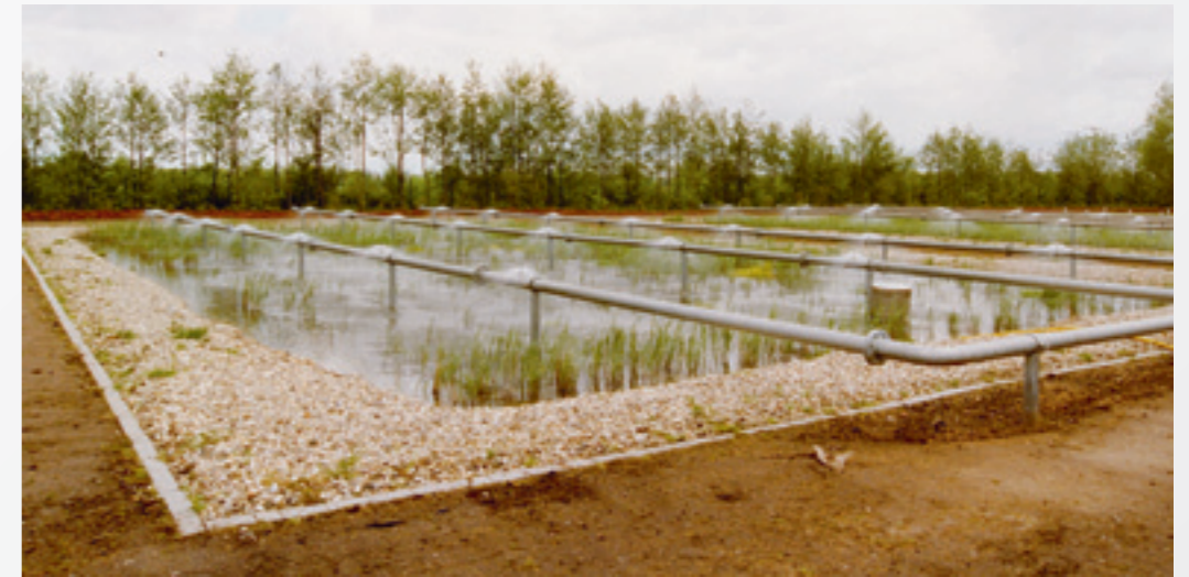
The constructed wetland in Sendenhorst allows surface water to be purified in a natural way.
